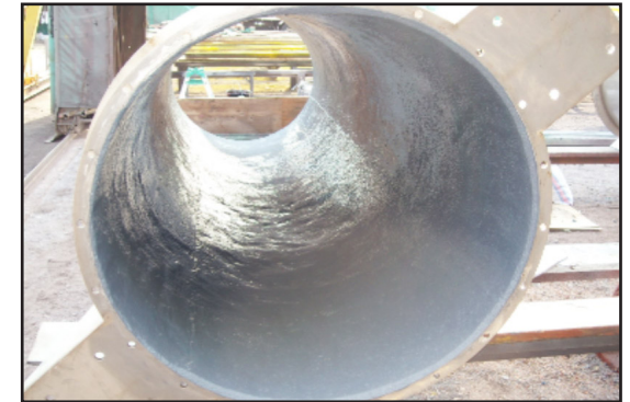
Finished section of the slag chute
